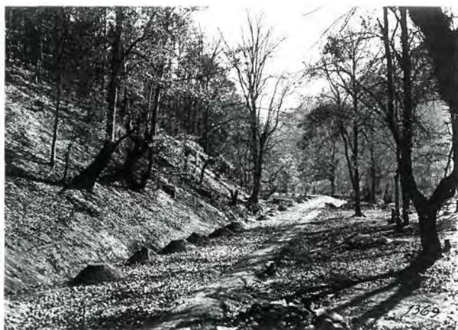
Slika 1. Šumska pruga u gradnji Figure 1. Forest railway under construction
